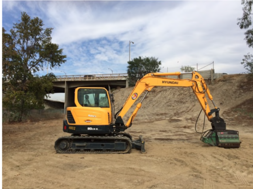
PHOTO 1: RUBBER TRCK EXCAVATOR WITH FLAIL MOWER
